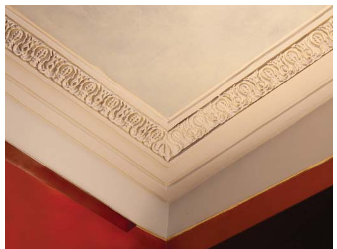
Detail of first-floor decorative scheme. Photograph: Lewis Bush
