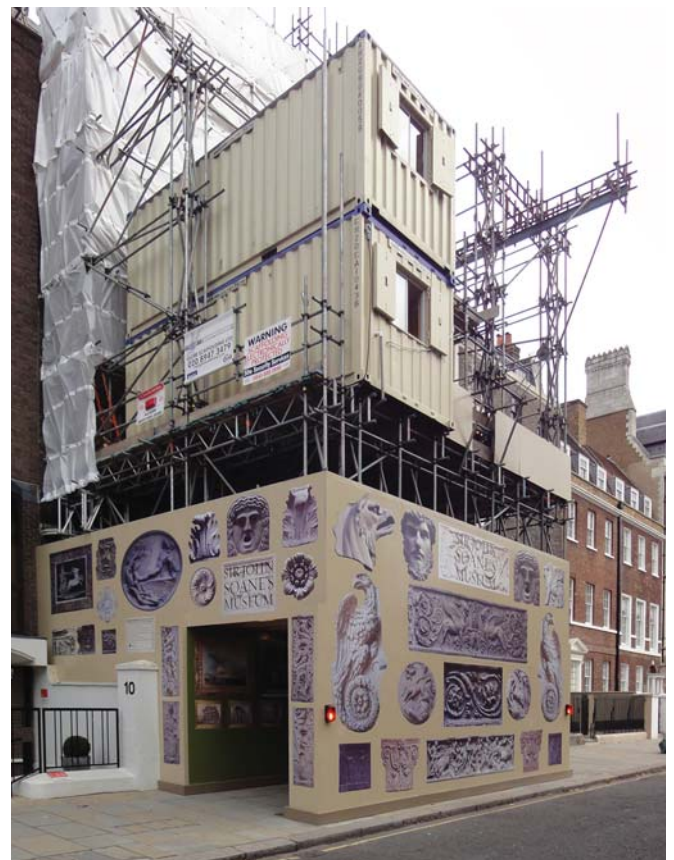
Scaffolding erected at the front of No.12. Photograph: John Bridges
